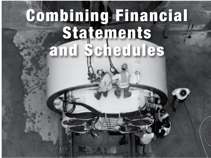
Bay Tunnel – Tunnel Boring Machine Assembly and Launch.
