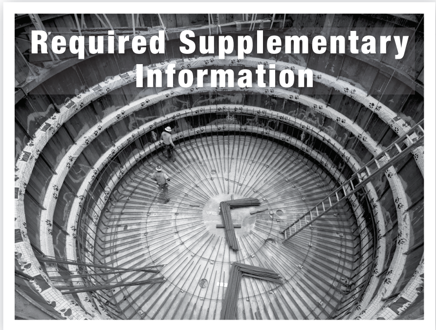
One of many new cisterns under construction. The new cisterns will enhance firefighting capacity throughout San Francisco.
