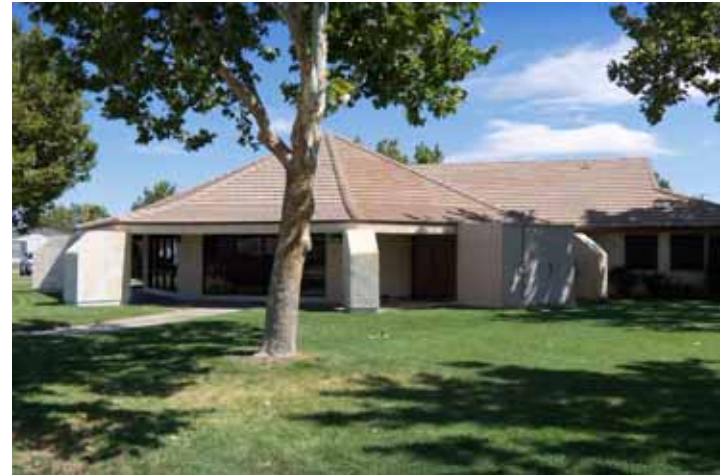
REAR OF RECREATION CENTER
