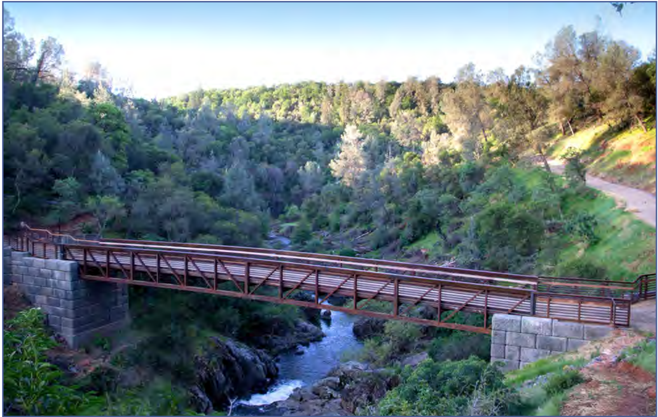
Hidden Falls Bridge
