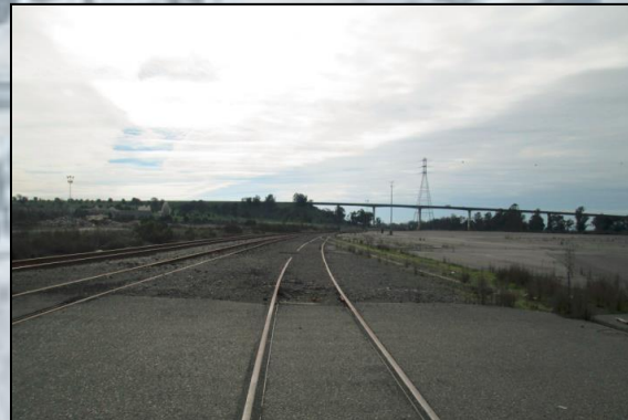
Looking south along the rail line
