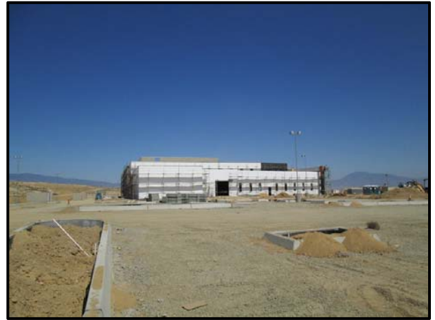
Looking east across the subject property
