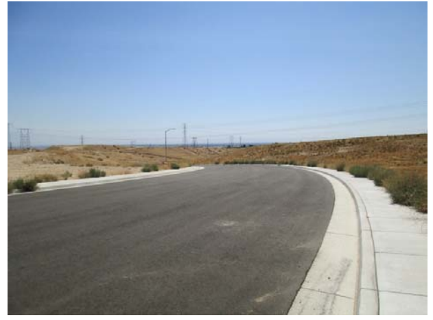
Highland Knolls Drive, south of transitional land
