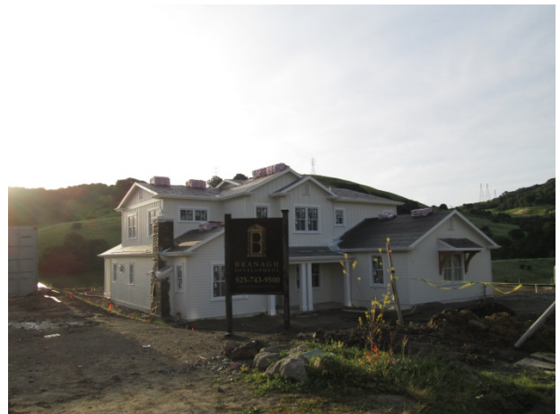
Home under construction – Frogs Leap Way
