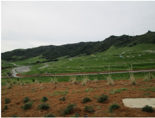
Southerly view across Wilder
