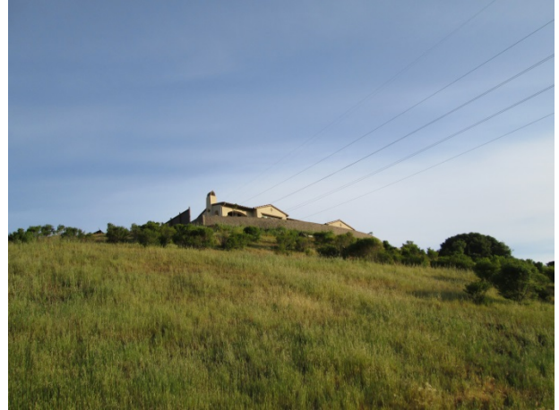
Looking northwest along Rheem Boulevard
