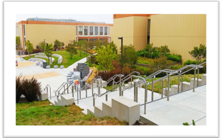
Skyline College Building 1 and 2
